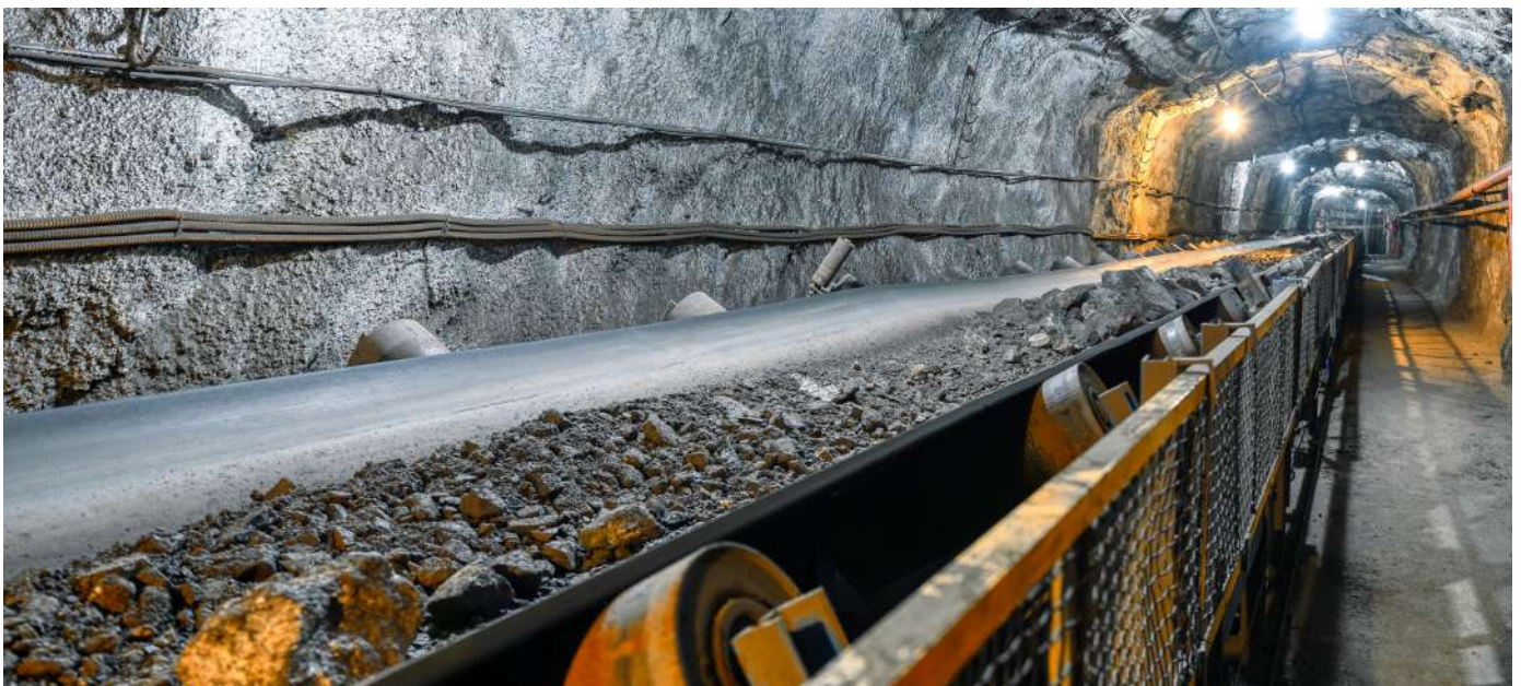
One of the applications of Flame Rock in an underground mine.
